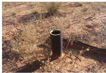
Plumbing would be replaced
